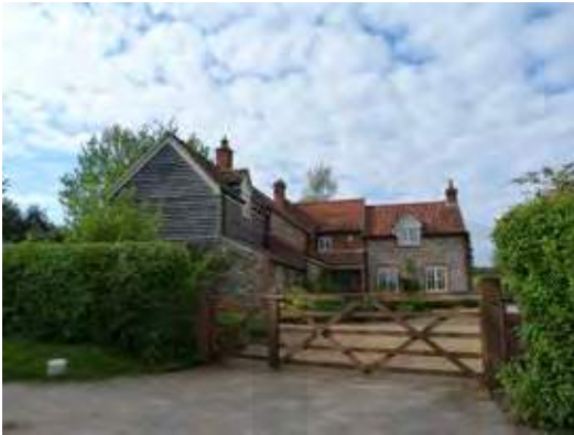
Modern side extension to an historic cottage in Stody
