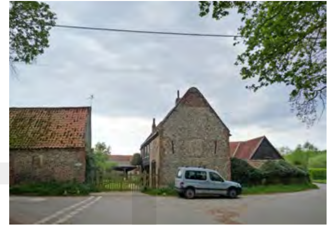
Converted agricultural buildings in Hunworth
