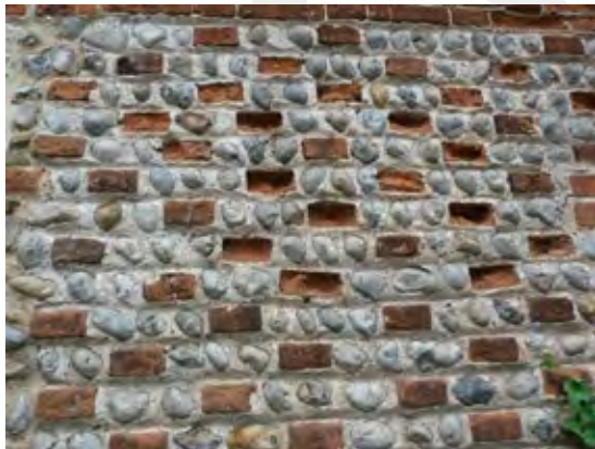
Cobbled flint and red brick patterning, with cement mortar
