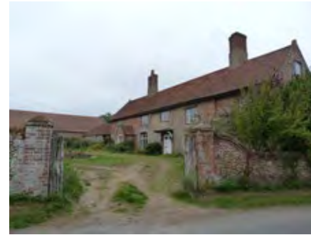
Farmhouse at Green Farm near Hempstead
