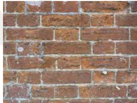
Red brick with lime mortar
