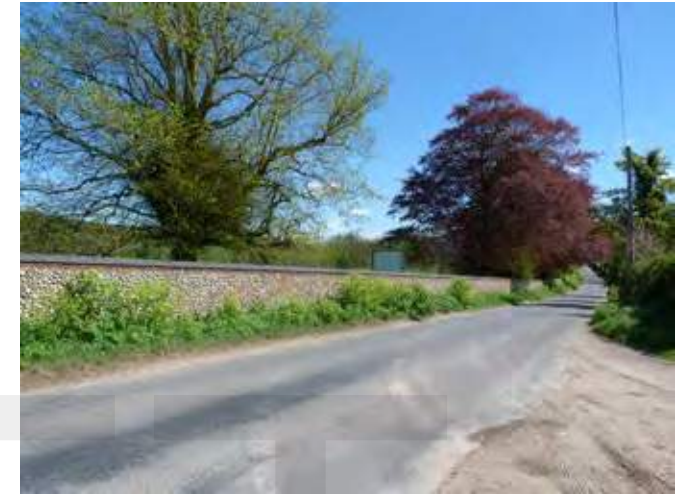
Wall bounding the Bayfield Hall site
