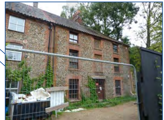
Hempstead Mill (also known as Holt Mill)
