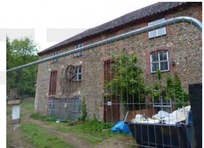
Hempstead Mill, which is vacant though there appears to be building work on the site. The building also has modern uPVC and timber windows that are out of character with the historic building and Conservation Area
