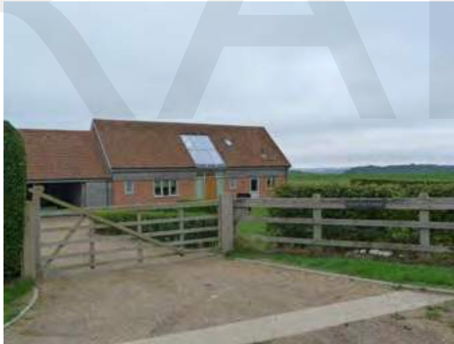
Timber cladding and glazing to a modern house near Holt
