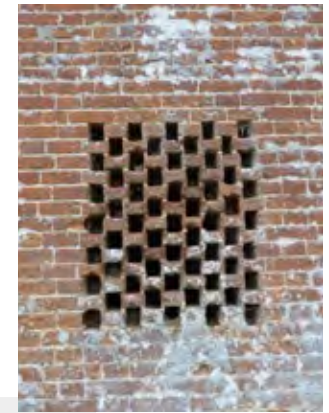
Red brick to a barn with ventilation detail
